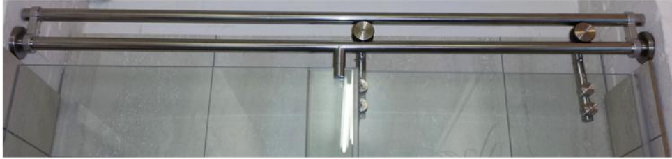
Fig.4 Completed view showing all sliding components in place
